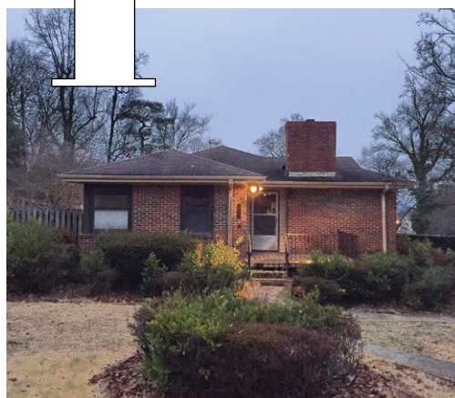
Built in 1949, the original structure had no style, says designer Doug Davis of Hannon Douglas. "It was dark, the window placement didn't make any sense, the front door was hidden, and the roofline was off."
